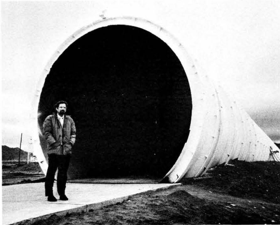
JIM NAKOS of Explosives Testing Division 7533 is the test project engineer. In the background is the 19-foot-diameter open end of the 520-foot-long high-strength steel tube.
